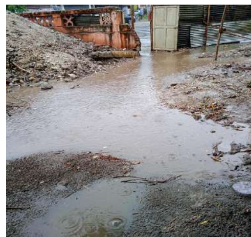
rainwater stagnation near main road
