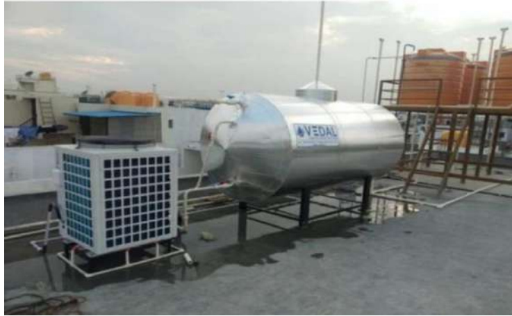
Diagram: Centralized Heat Pump Water Heater
