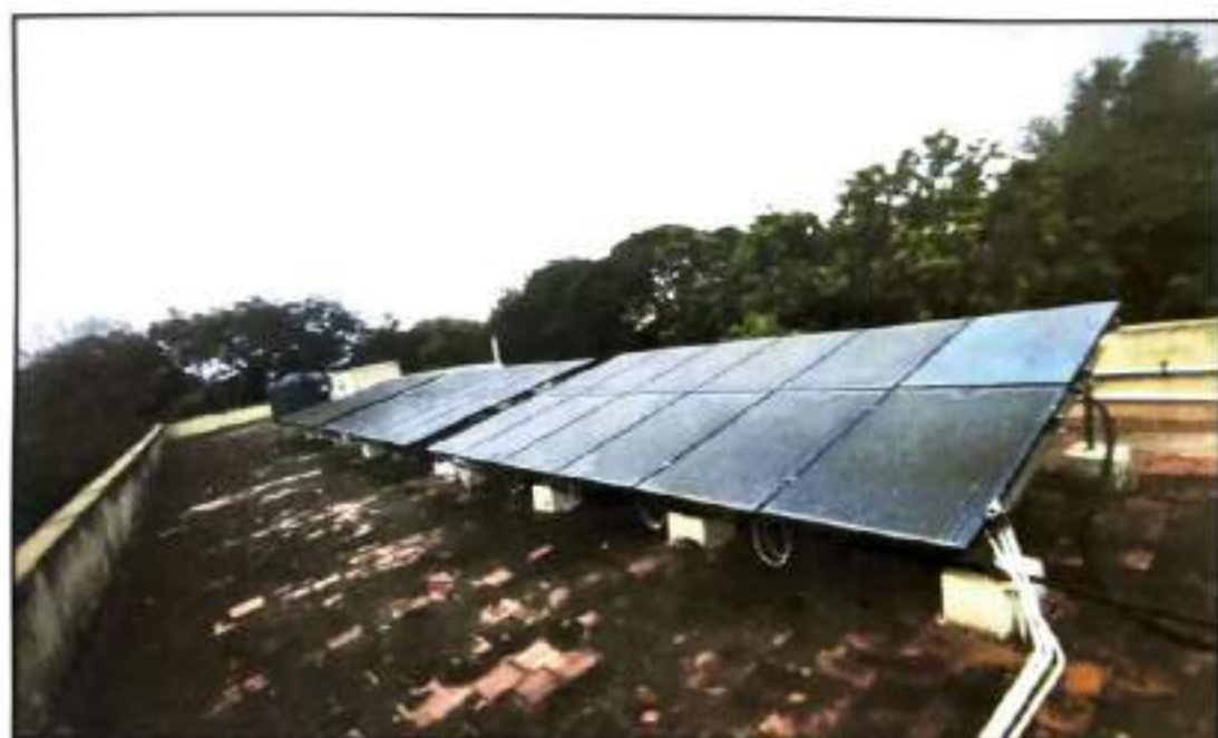
Solar Unit in Government College of Technology, Thadagam Road, Coimbatore, Tamil Nadu
